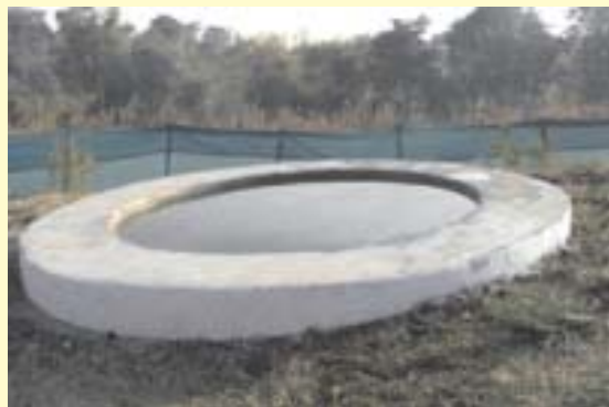
Water storage tank in nursery
